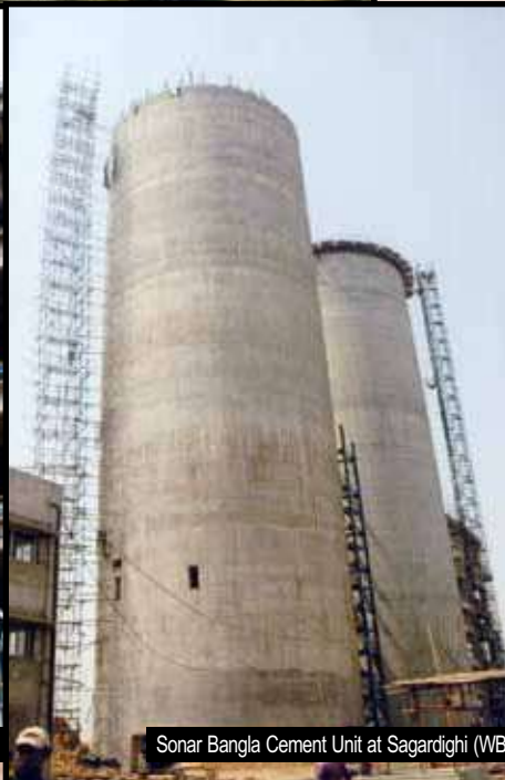
Cement Storage Silo for Penna Cement Ind Ltd. (AP)
